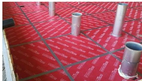
Seal the horizontal and vertical joints carefully with the Stik tape.
